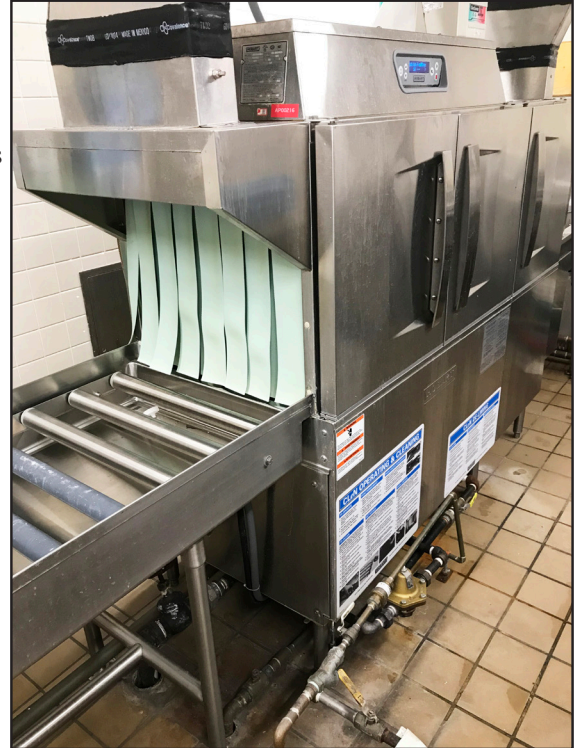
NVRH Food Service replaced the 45 year old dishwasher in 2017. The new model is Energy Star® rated and has an energy recovery system that captures escaping heat and steam from the exhaust and recycles it into free energy that preheats the incoming water supply.
